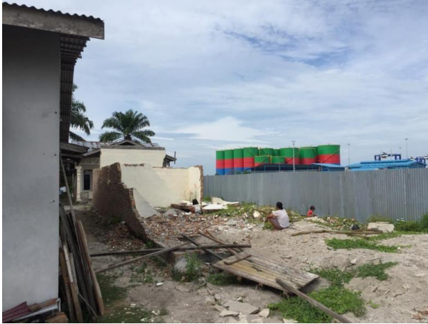
Fig.3 Residents' Houses Affected by Road Construction to TCC
